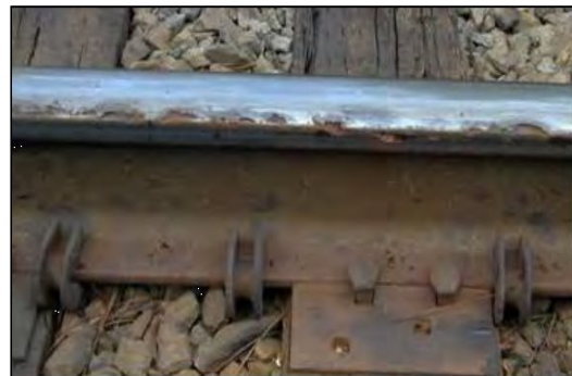
Severe Shelling Gage Corner
