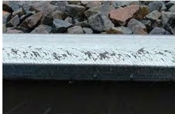
Severe Checking with Spalling
